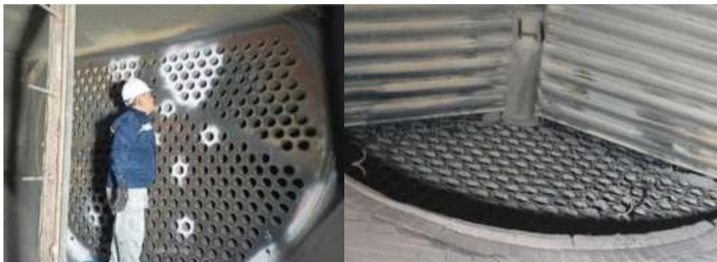
Figure 5 (A). East side of the Pipe Plate and (B) The West side of the pipe plate is filled with crust from combustion residue.
