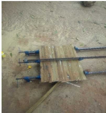
Figure 2: Fabrication of the glulam
